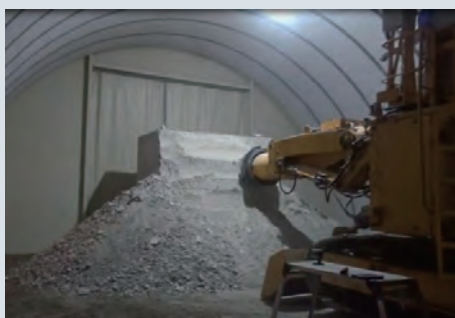
Fig. 3. Excavation verification at simulated tunnel test site
